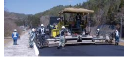
Pavement recycling technology
